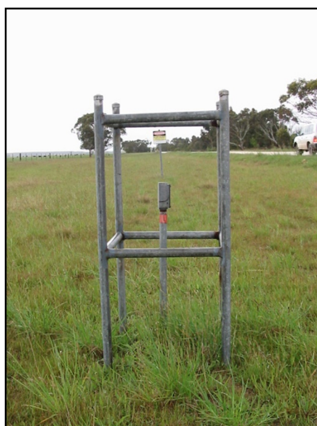
Plate 5 and 6: Cathodic Protection Test Post and Pipeline Marker Sign
