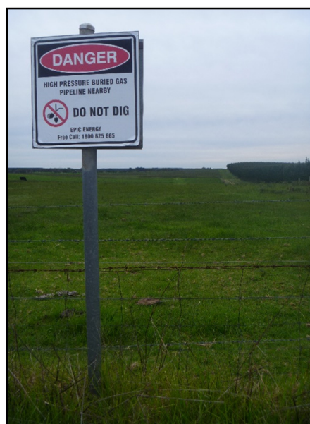
Plate 5 and 6: Cathodic Protection Test Post and Pipeline Marker Sign
